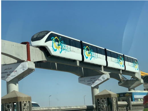
New Administrative Capital Monorail Project in Cairo
